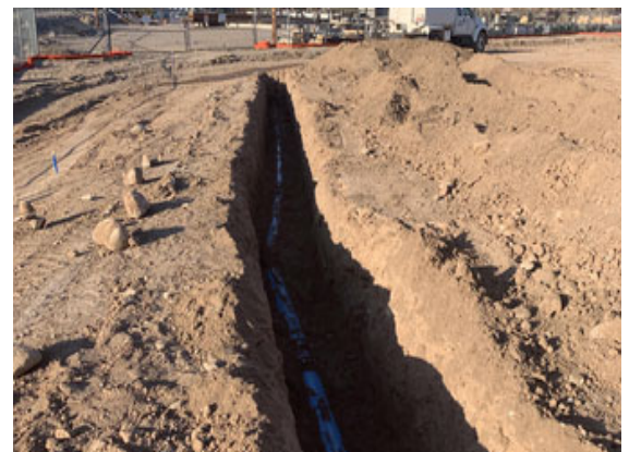
East fire line being installed 7/26/19
