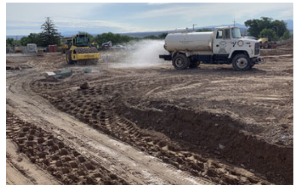
Building earthwork compaction 6/10/19
